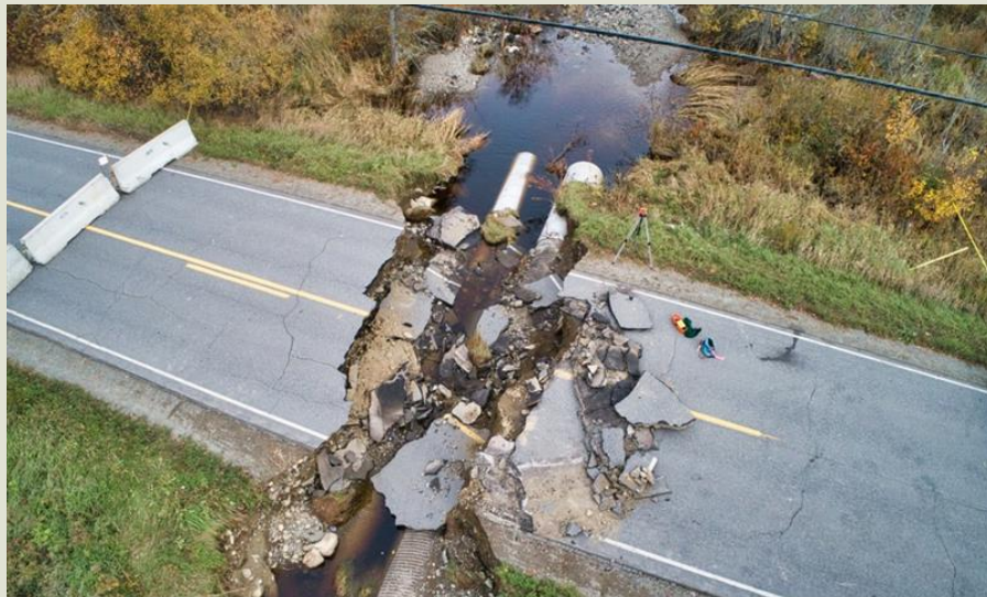
Culvert washout on Pushaw Rd in Glenburn, ME in October 2022 associated with a 25-year storm event. The washout resulted in a 5-mile detour and cost $111,000 to repair.
