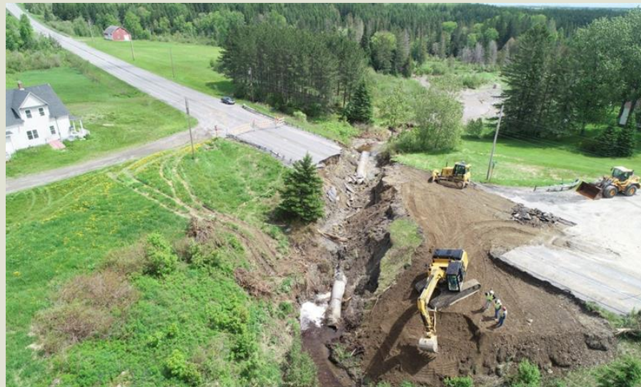
Culvert washout on Route 1 in Cyr Plantation, ME in May 2022 associated with a 50- to 100-year storm event. The washout resulted in road closure and detour and cost $2.8 M to repair.
