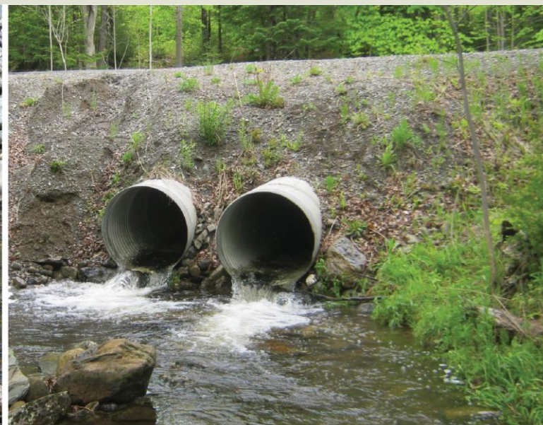
Culvert washout on Route 1 in Cyr Plantation, ME in May 2022 associated with a 50- to 100-year storm event. The washout resulted in road closure and detour and cost $2.8 M to repair.
