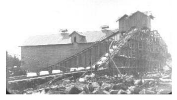
Figure 3: Ice blocks moving from the pond to the storehouses.
